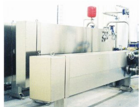
Heat exchanger sludge/water and heat exchanger unit sludge/sludge from Läckeby installed in Älmhult, Sweden
